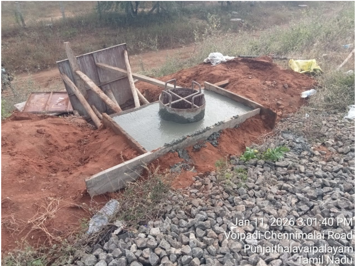
420/40 BG7, CONCRETE WORK ON GOING
